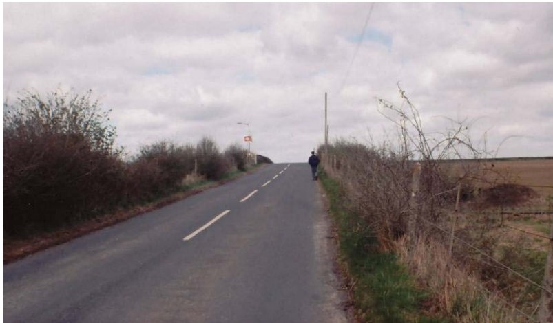
Figure 7.1: Thornford Station: poor access
